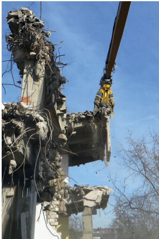
The lightweight Concrete Busters are ideal for high reach deconstruction. Perfect for demolition sites in residential areas.
